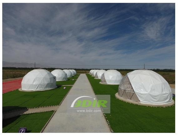
In June 2017, BDiR Inc. received a project to build a dome tent hotel in Qinghai Resort. Through field trips, which combined with the local desert environment, 12 semi-permanent spherical dome tents were designed and built. Because of the temperature difference between day and night, the spherical dome tents are selected to match the elastic cloth and insulation cotton to improve the warmth of the tents and ensure that the temperature inside the tent is moderate.
