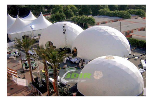
The use of galvanized and white printed steel tubes makes the entire dome structure more lustrous and durable, with better rust and corrosion resistance and a long life of 30 years. The 850 g/m2 PVC fabric membrane is with the function of UV, water and tear resistance. As a professional event dome manufacturer, our PVC fabric membrane meets European (DIN4102 B1 M2) and US (NFPA701) flame retardant standards.
